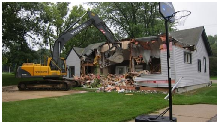
Demolition of the grey house. September 2014
